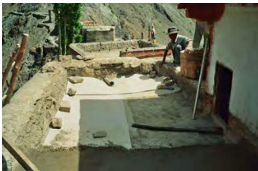
One particular problem during refurbishment was that the thickest – and thus heaviest – layer of the roof was resting on a relatively delicate ceiling structure, as evidenced by visible water damage inside.
