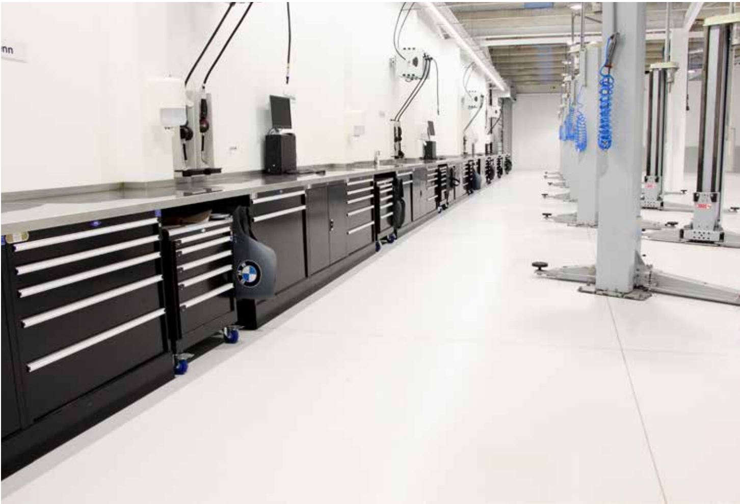
New Zealand Specialised Coatings is New Zealand's largest Sika approved applicator and has a wealth of experience in applying specialised flooring systems. NZSC used Sikafloor-264 with Sikaglaz PU for this quality project.
