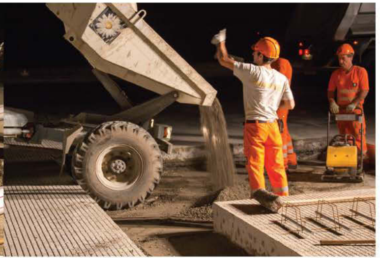
A good sense of proportion comes handy for estimating the lean concrete needed.
