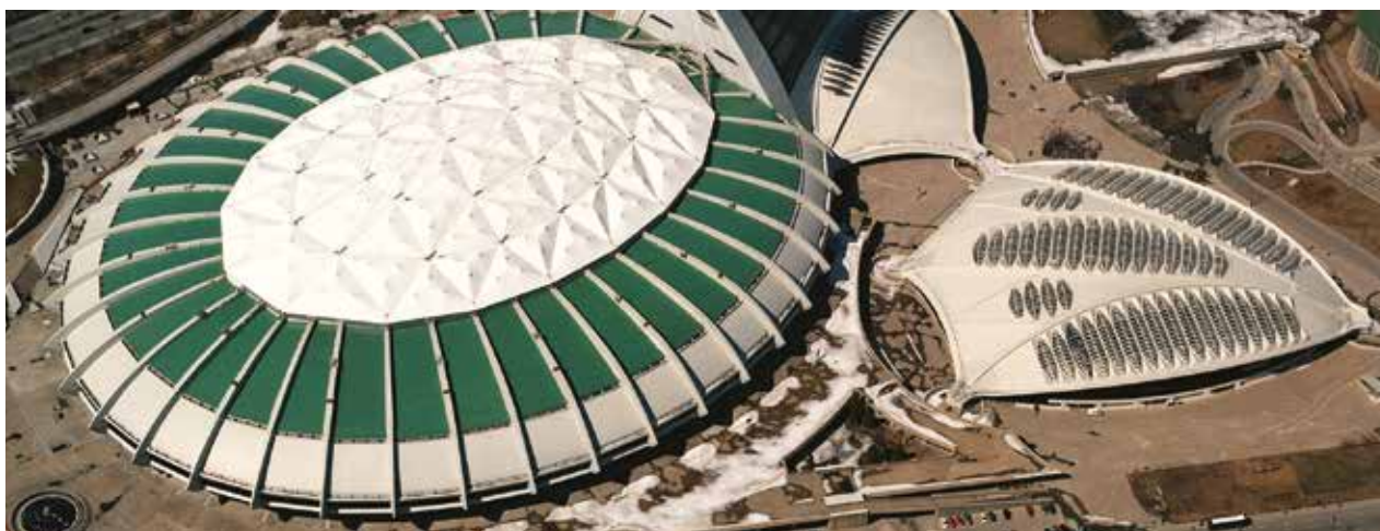
Olympic Stadium, Montreal, Canada
