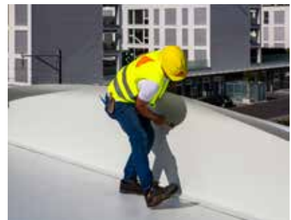
3. Sarnafil® AT FSA P Bahn anbringen
