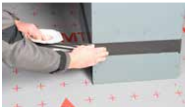
SikaRoof® Tape 60 Weld anbringen.
