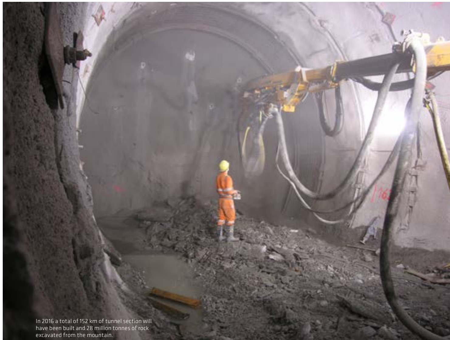
Challenging demands for the tunneling engineers: high underground temperatures of 30 to 40°C had to be managed.
